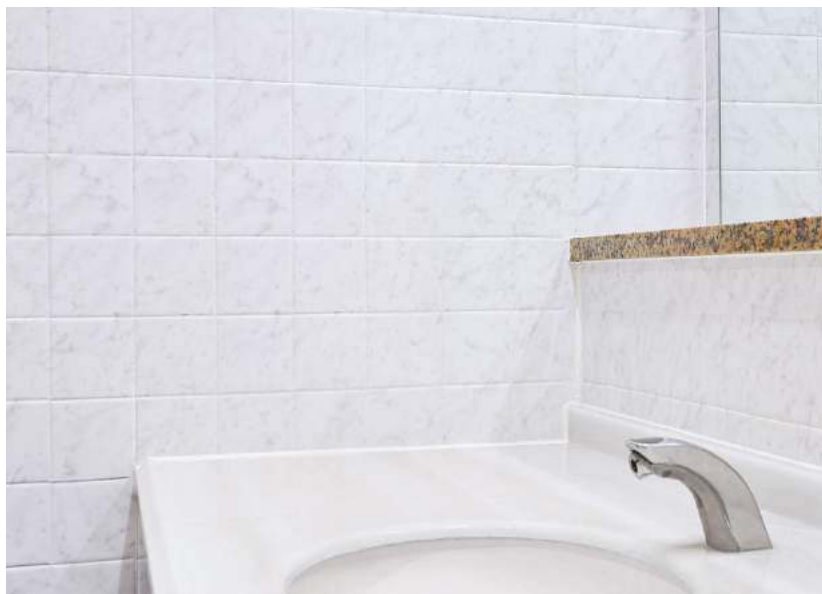
Restroom refurbishment / ST-024TIL
