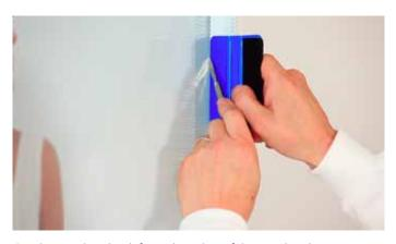
Cut the graphics back from the edge of the window by 1-3mm to ensure reliable edge adhesion.
