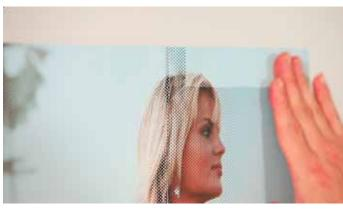
Take the second panel, cut away the top 25-50mm of the liner. Align the design of the first and second panels, applying second panel with overlap.
