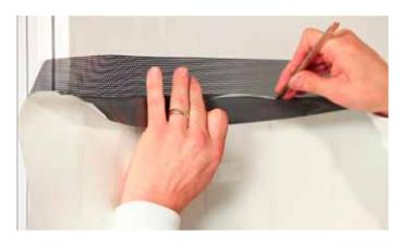
Apply dry using a plastic applicator with a low friction sleeve. Avoid touching the adhesive, especially at the edges and corners. Cut away the top 25-50mm of the liner.
