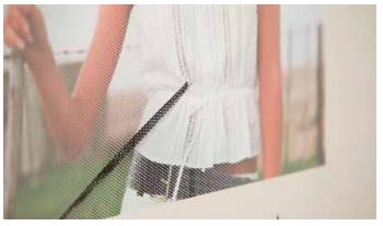
Remove the trimmed excess film to form a clean butt join.
