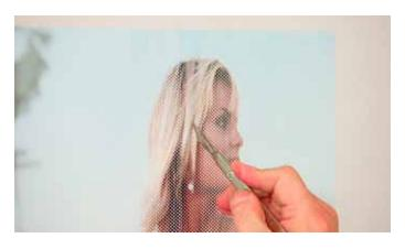
Cut down the centre of the overlap, through both layers of material taking care not to scratch the glass.
