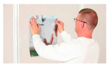
Use a butt join, not an overlap join. Apply the first panel.
