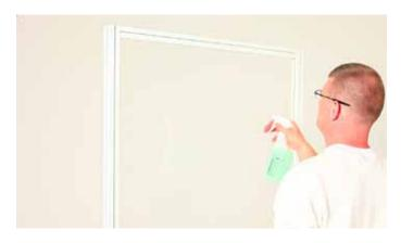
Surfaces to which the material will be applied must be thoroughly cleaned from dust, grease or any contamination that could affect the adhesion of the material.
