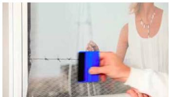
Otherwise, just squeegee down evenly, handling the graphic with care, and ensuring that no bubbles are trapped beneath the graphics.
